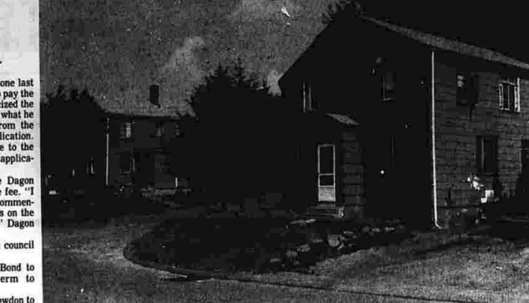
Inspections of 450 housing units at Mayberry Village revealed no major housing code violations. The units which were inspected are in the older section of Mayberry Village. The section was built as a public housing project for the families of soldiers during World War II. The town later sold the projects. (Herald photo by Blake)
